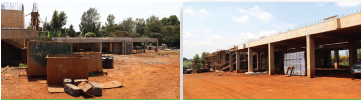
Figure 12: The Miran Residence Construction Progress
